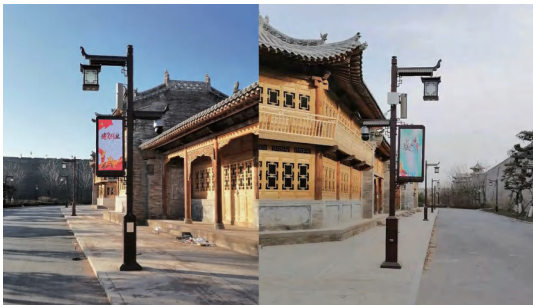
Smart pole project Location: Shanxi
