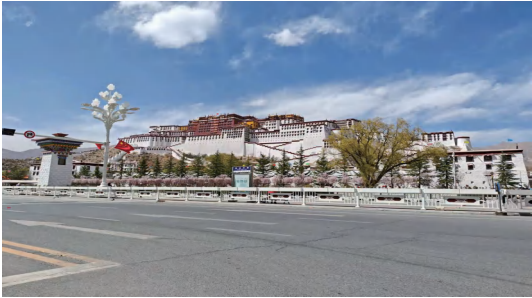
Smart Street lighting project Location:Lasa | Quantity:40,000+
