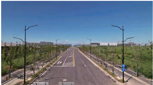
Smart Street lighting project Location:Shanghai | Quantity:40,000+
