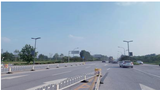
Smart pole project Location: Xiongan
