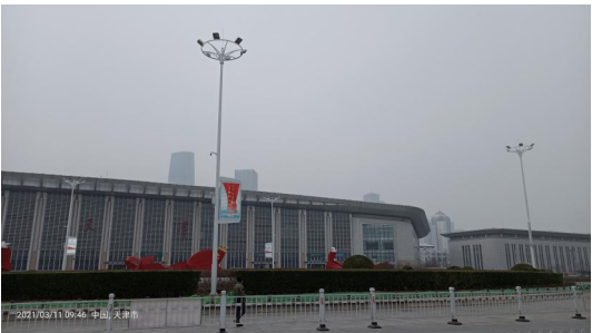
Smart Street lighting project Location:Tianjin | Quantity:27,000+
