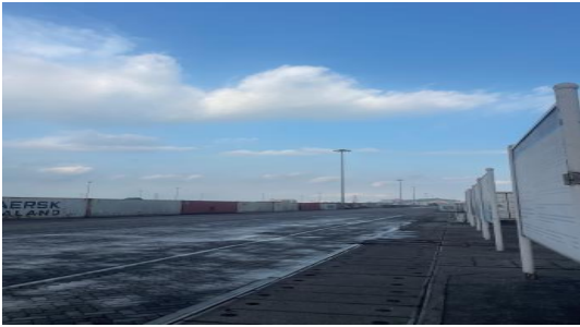
Smart port lighting project Location: Putou port in Putian
