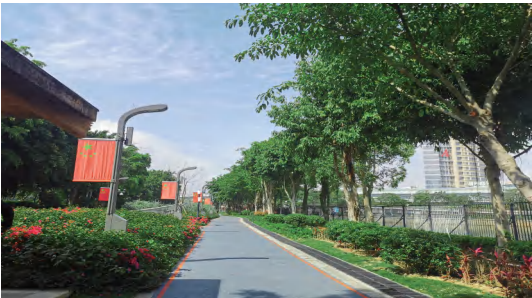
Smart Street lighting and Smart Pole Location:Xiamen
