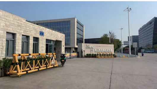
Smart port lighting project Location: Haitian port in Xiamen
